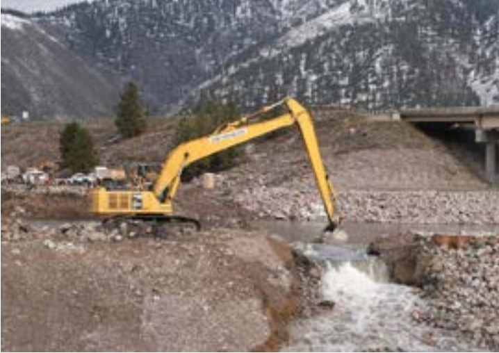
An Envirocon excavator at work.
