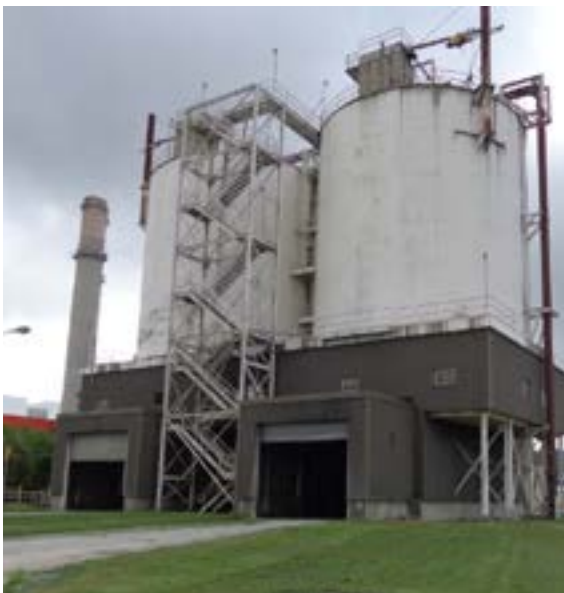
Coal ash silo at a large power generation facility.
